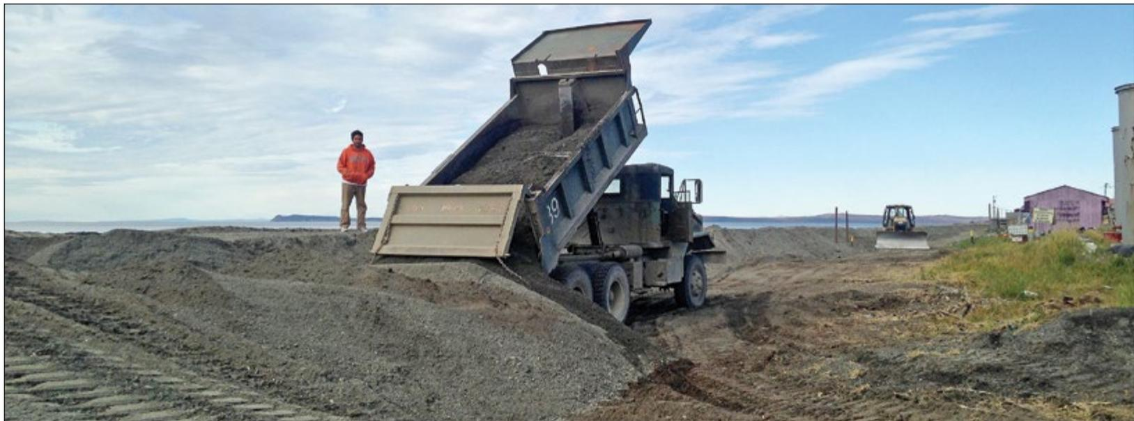
*Workers build an earthen berm to help prevent flooding.
