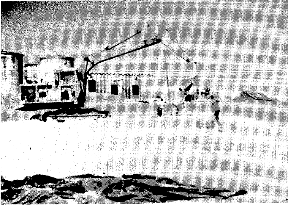
13. Noatak, Pumping Grout into ARMORFORM
