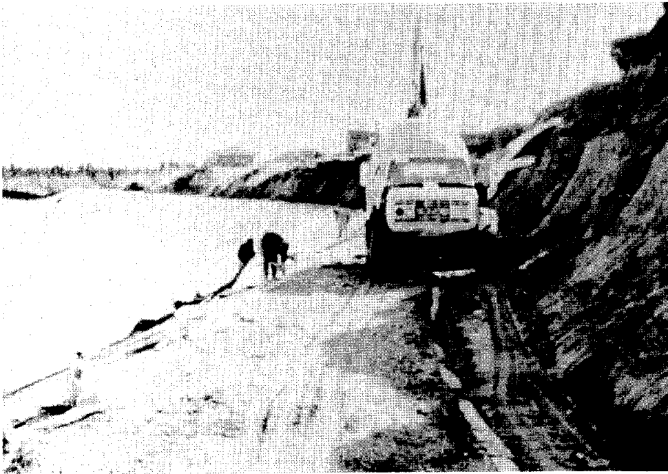
14. Noatak, Pumping Grout into ARMORFORM
