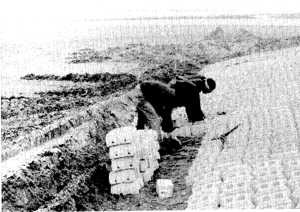
4. Hooper Bay. Stringing the ARMORFLEX Mattress by Hand
