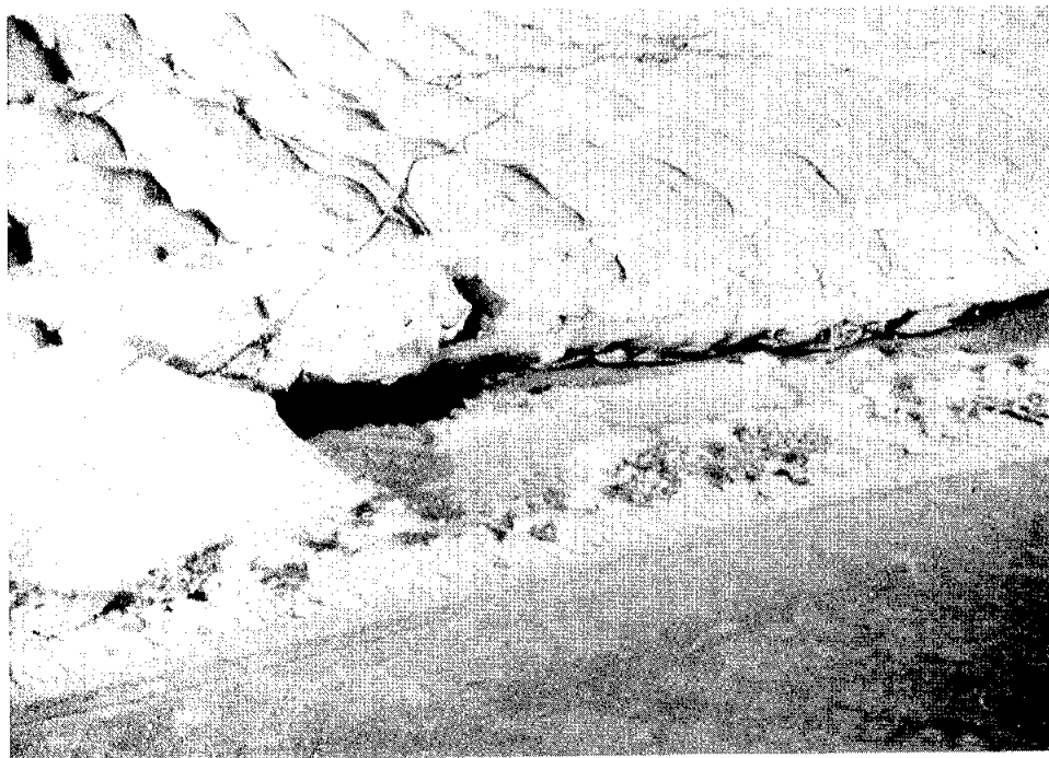
20. Noatak, the ARMORFORM has Slipped Down Slope
